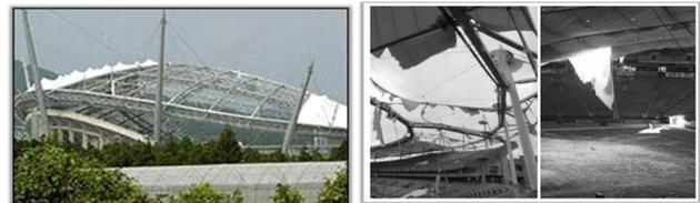
Fig. 2. Membrane defect case
