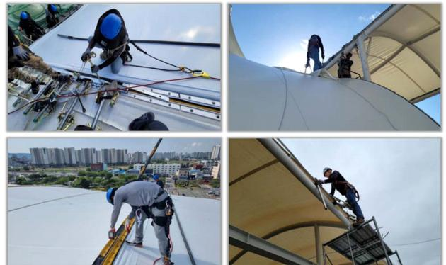
Fig. 1. Case of roof membrane pulling construction work
