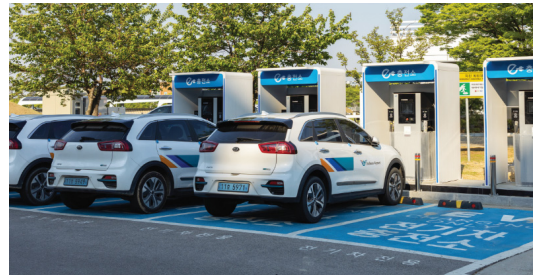
Fig. 2. Electric vehicle charging station at ICN
