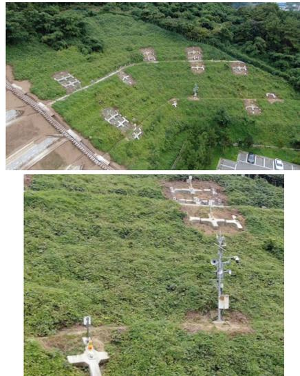
Fig. 7. Landslide detection sensors installed on-site
