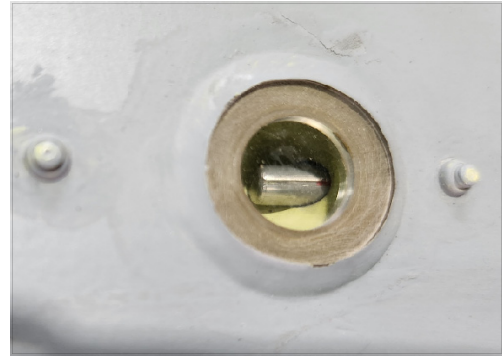
Fig. 19. Appearance of the applied inspection window
