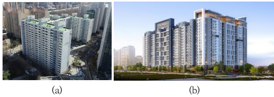
Fig. 10. Views of Sinbanpo The Sharp Riversky [15,16] (a) Before Remodeling (b) After Remodeling
